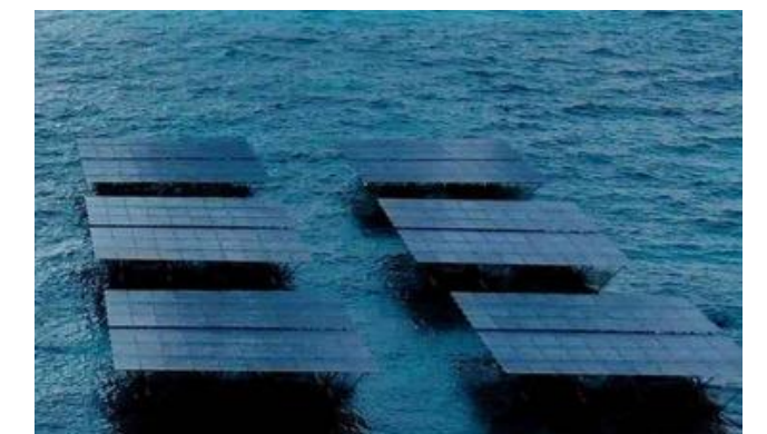
Systems ranging from 12 kWp to 427 kWp, operating nearshore in Maldives – Swimsol
